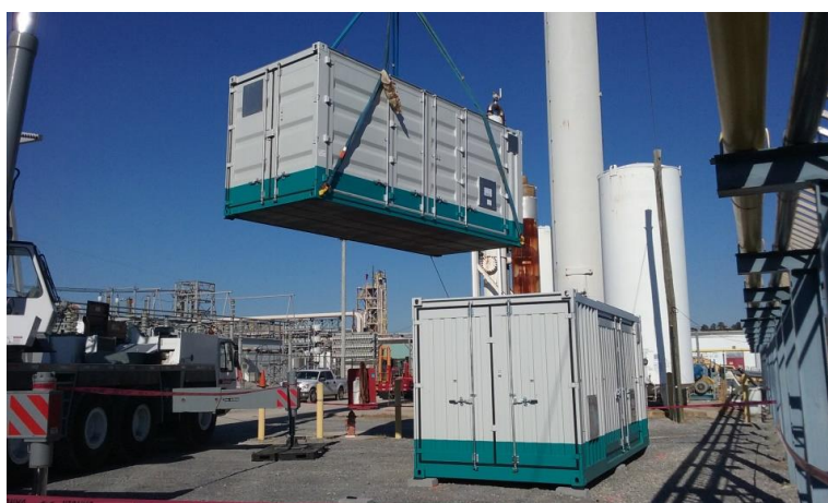
Delivery of the Liquid Organic Hydrogen Carriers (LOHC) applications at the United Hydrogen Group (Tennessee, USA). (Photo: Hydrogenious Technologies GmbH)
